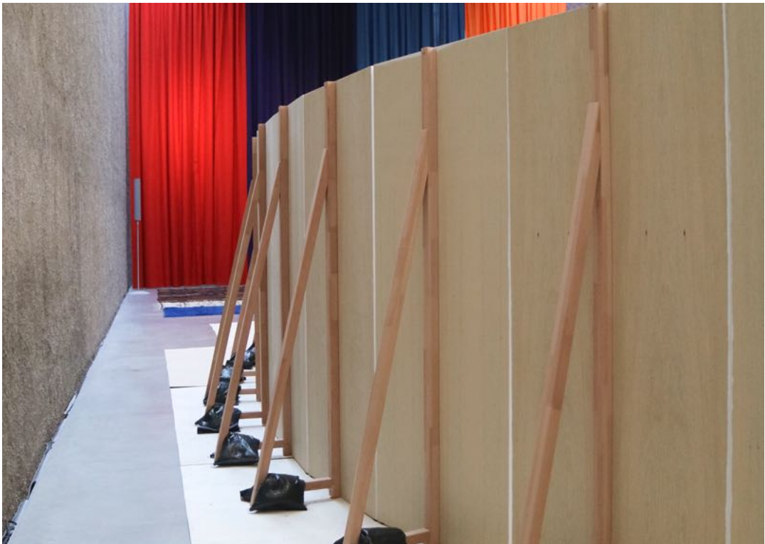
Example of lightweight door blanks with wooden A-frame and sand bags
